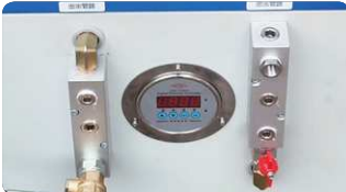
Quick water pressure testing
